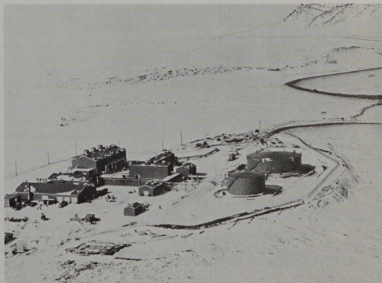
Pump Station 4, located in the northern foothills of the Brooks Mountain Range, is accessible by the road the BLM pipeliners travel.
